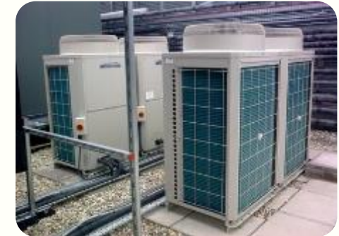
More than 90% of AC used are efficient VRF
