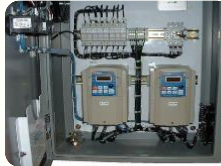
100% of SEU : VFD control & Idle time eliminated
